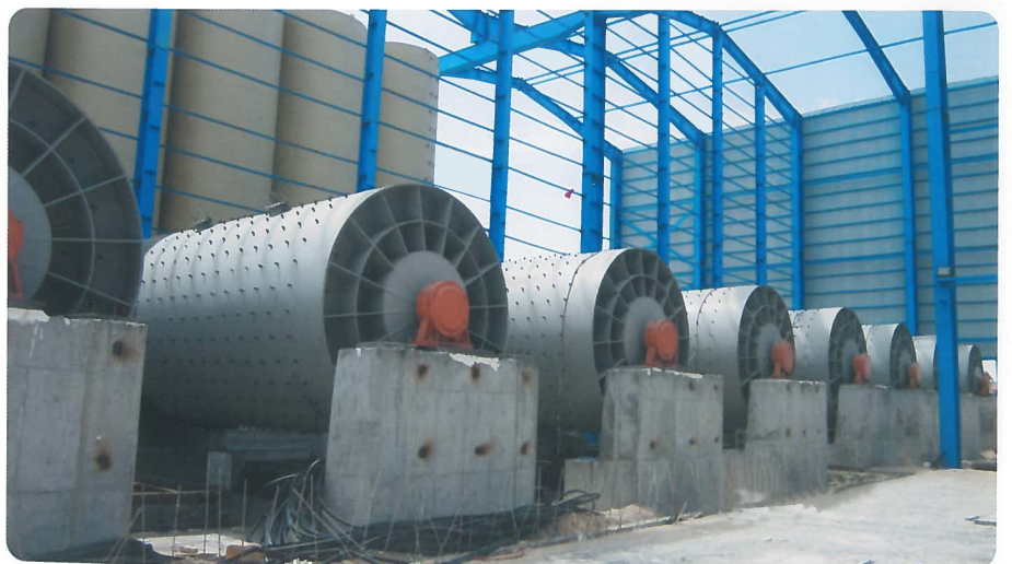
Assembling Site In The Factory
